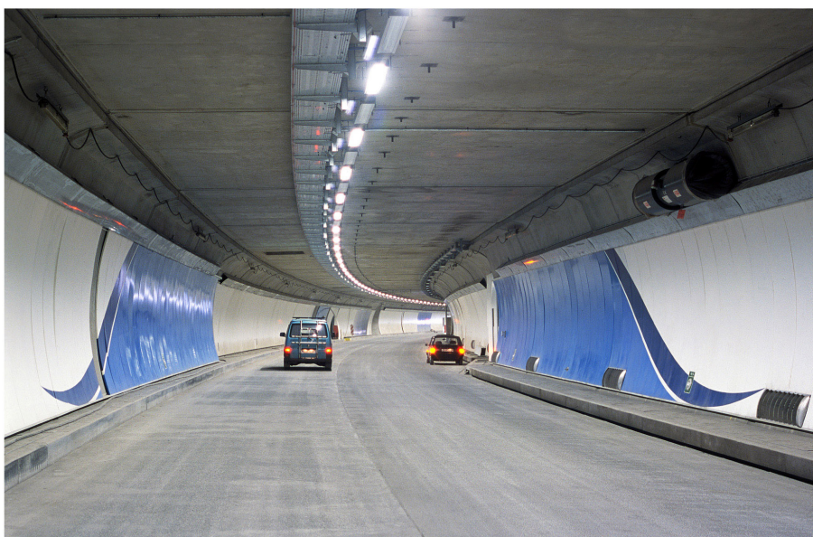
© photo-daylight.com, Copyright free for all publications edited by CEMBUREAU/BIBM/ERMCO Members including web sites Cointe tunnel (link E25-E40) in Liege, Belgium: use of concrete road pavement for improved tunnel safety
