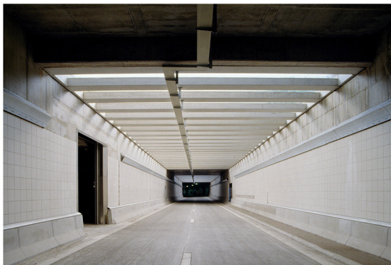
© photo-daylight.com, Copyright free for all publications edited by CEMBUREAU/BIBM/ERMCO Members including web sites Kinkempols Tunnel (link E25-E40) in Liege, Belgium, using concrete pavement
